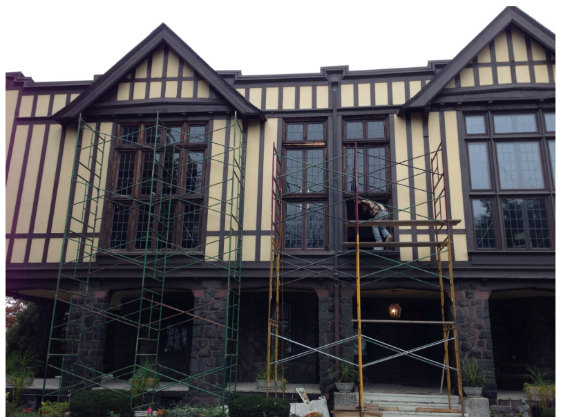
Hard at work on window restoration!
